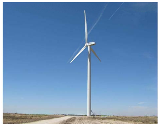
The installed D8.2 at Sweetwater
