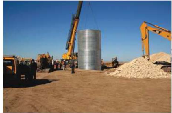
Installation of Outer Can of the foundation
